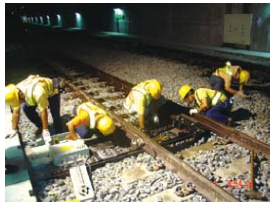
號誌隊號誌電動轉軌器附件間隙調整
