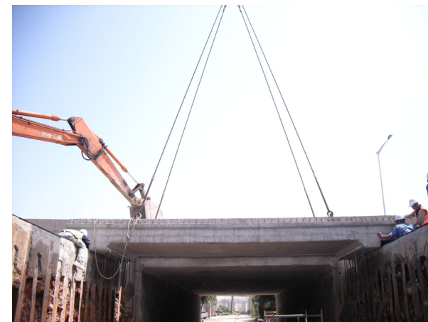
半逆打預鑄頂版吊裝
